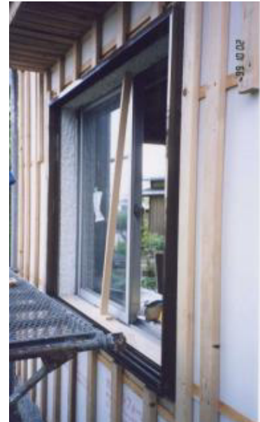
Figure2 Enveloping with insulating material and an additional window sash
