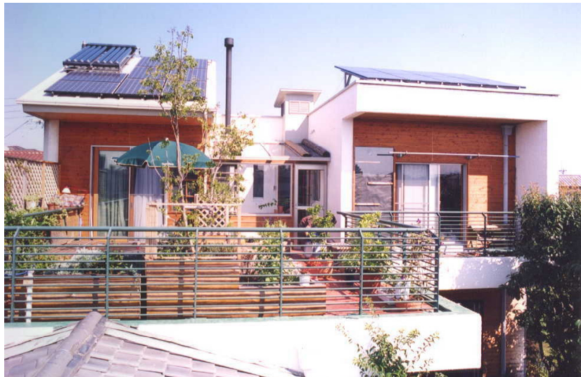
Figure5 Building appearance after renovation, south facade
